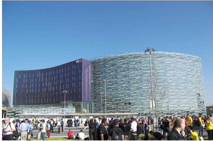
Office building, London, United Kingdom
