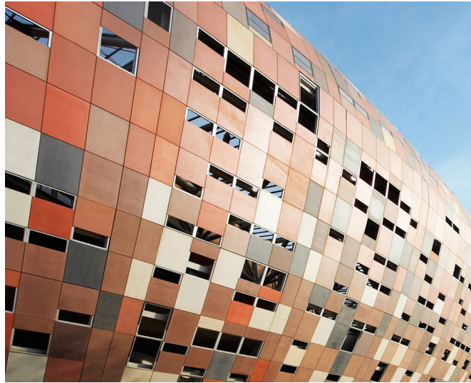
Fiberglass-concrete facade, „Soccer-City”, Johannesburg, South Africa
