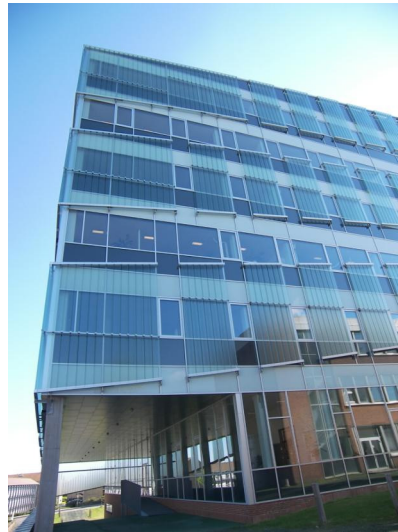
U-profile glass facade system, VIA University College, Horsens, Denmark
