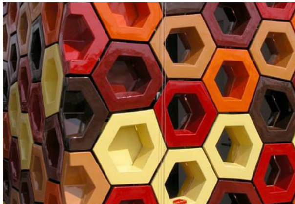
Ceramic facade covering, Spanish Expo-Pavilion, Aichi, Japan
